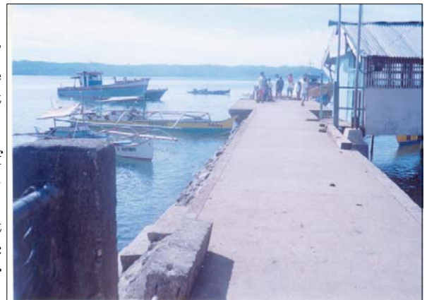
Municipal Fish Port of Sarangani: Port component of the Infrastructure Support to the Economic Program of Sarangani, Davao del Sur
